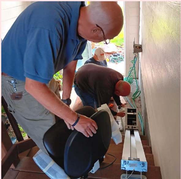
Installing Sylvia Kimbley's electric chair lift Photo by Beth Kidwell
